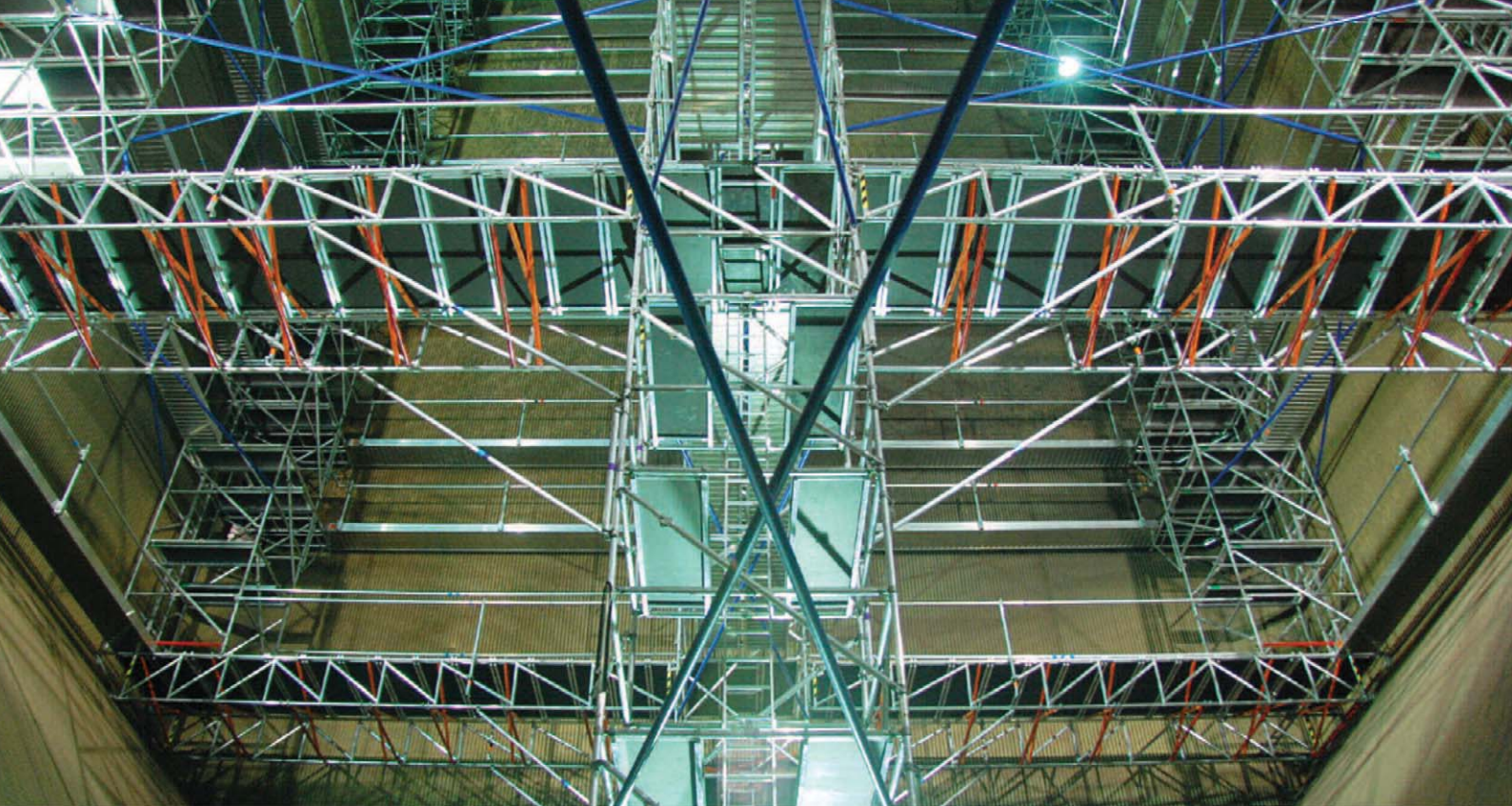
Above: Manjung Boiler Access System, Malaysia 660MW unit commissioned in November 2007. View looking from the bottom of the hopper showing base trusses and upper structure.
