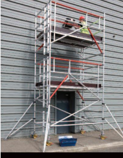
Instant AdvanceGuard is a new integral advance guardrail system that provides total fall prevention for the operator throughout assembly and dismantling of the tower.
